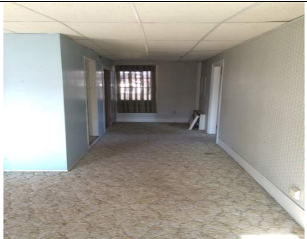
HM# - 23 2'x4' Dots and Gouges Suspended Ceiling Tile HM# - 24 Drywall and Joint Compound
