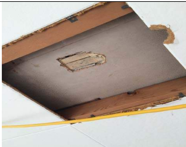
HM# - 2 Ceiling Plaster with Wall Coverings
