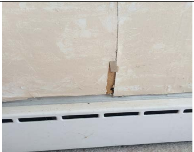
HM# - 21 Skim Coat over Particle board
