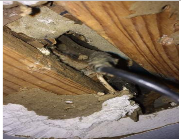
HM# - 10 Loose fill Vermiculite Insulation
