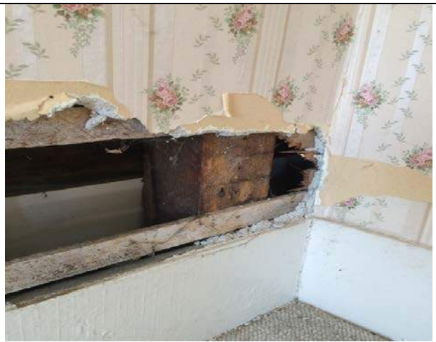
HM# - 1 Wall Plaster with Wall Coverings
