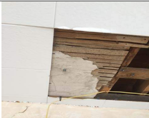
HM# - 7 12"x12" Tongue and Groove Ceiling Tile
