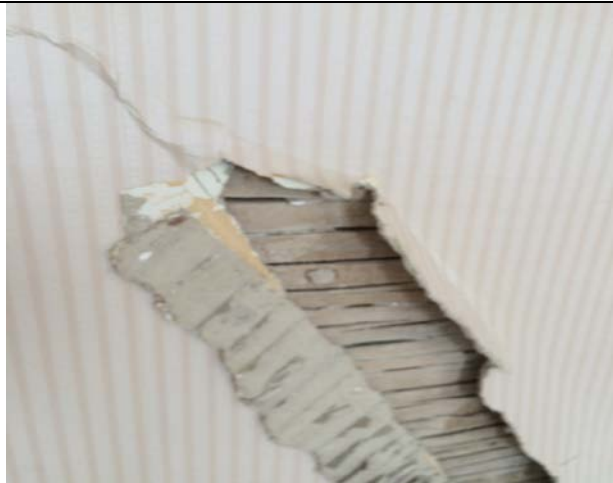
HM# - 16 Wall Plaster with Wall Coverings
