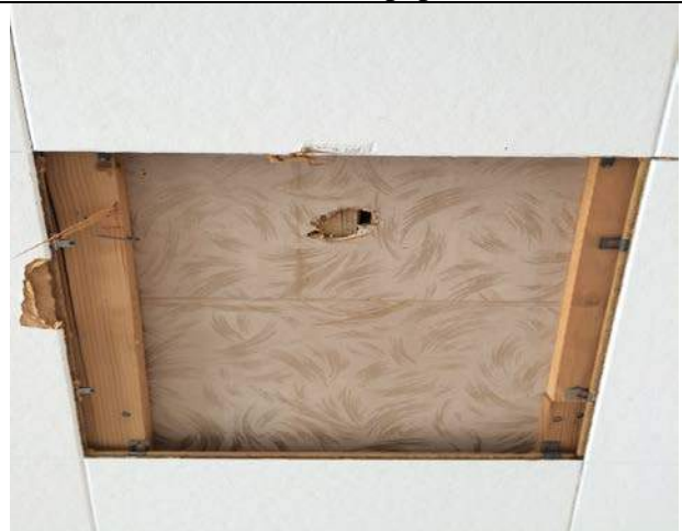
HM# - 17 Ceiling Plaster with Wall Coverings
