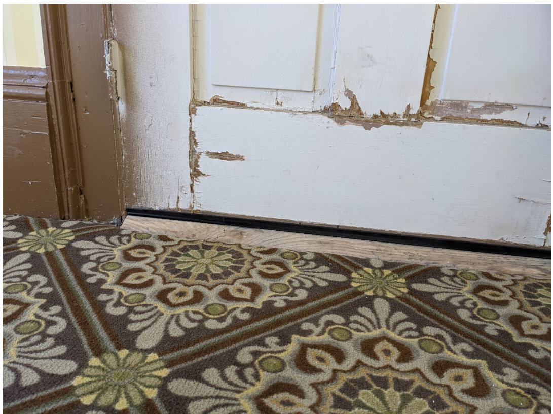
Verification Photo – Gasketing added to bottom of door.
