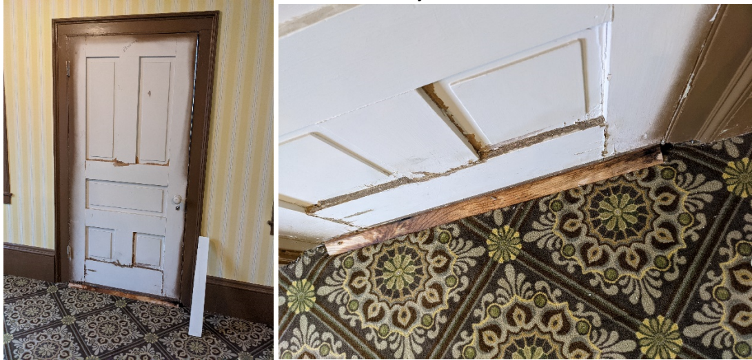
Verification Photo – Gasketing added to bottom of door.
